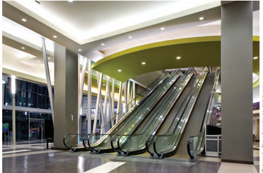
World Market Center in Las Vegas, Nevada, uses over 8,000 ft (2,438.4 m) of eW Cove Powercore linear LED lighting fixtures from Philips Color Kinetics to illuminate the complex geometries of the atrium in its Building C. LED cove lighting offers advantages over conventional cove lights in high-end installations such as this one. With useful life of up to 70,000 hours, and a very low failure rate, LED cove lights virtually guarantee reliable illumination around the clock for many years, without dark spots from lamp outages that can mar the elegant and uniform presentation of a premier space.
